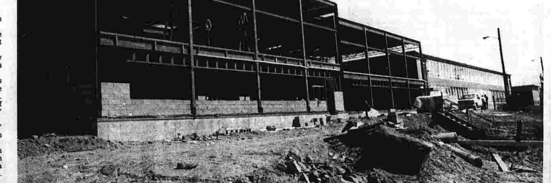
Iling Addition Begins to Take Form
